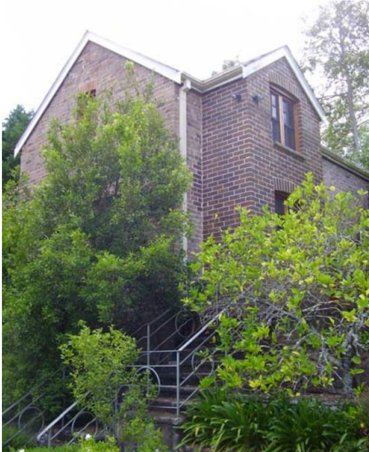
Image 1: Former “Lanosa” stables at 11 Kywong Avenue, Pymble
