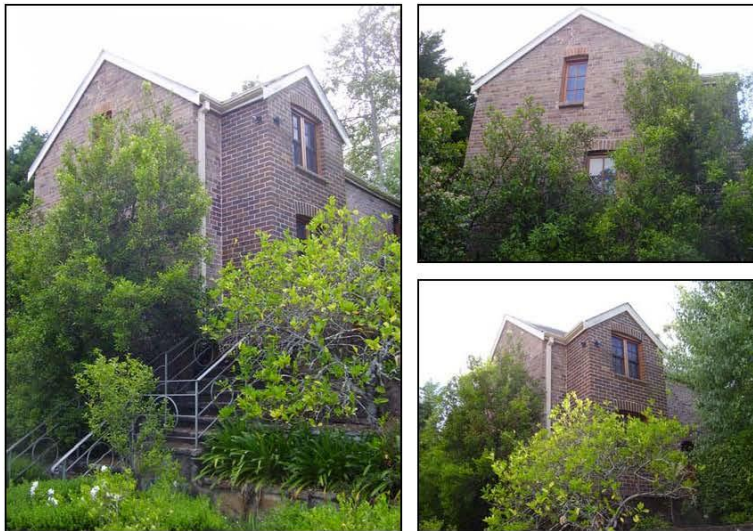
Former Stables No. 11 Kywong Avenue, Pymble
