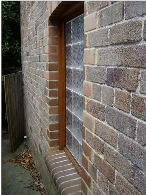
Figure 3.13 The glass block filled opening on the eastern façade.
